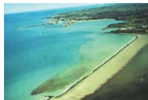
Outfall with Shoreline Impact
